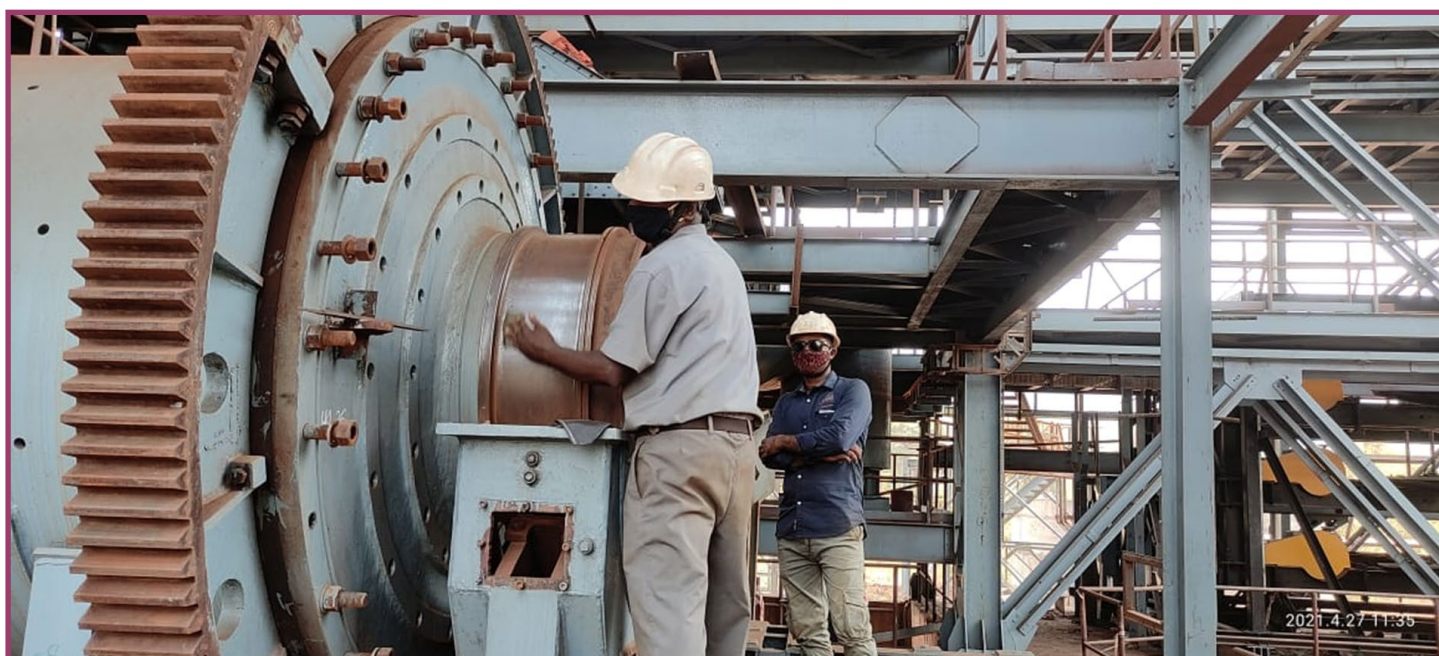
[Erection of Rod Mill in progress at OMC at South Kaliapani]
