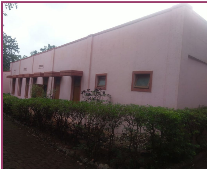
[Renovated School Building]
