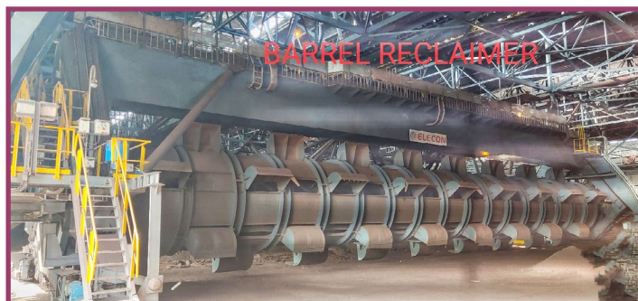
[View of Blender Reclaimer]
