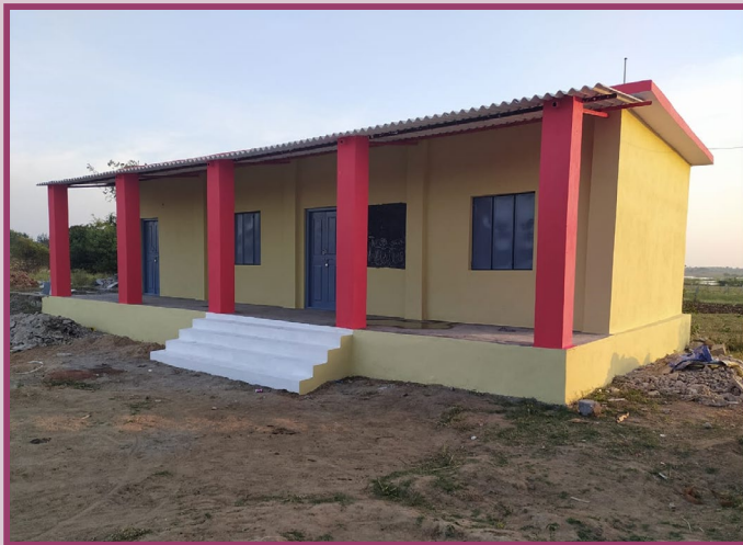
[Two Class Rooms constructed by KIOCL]
