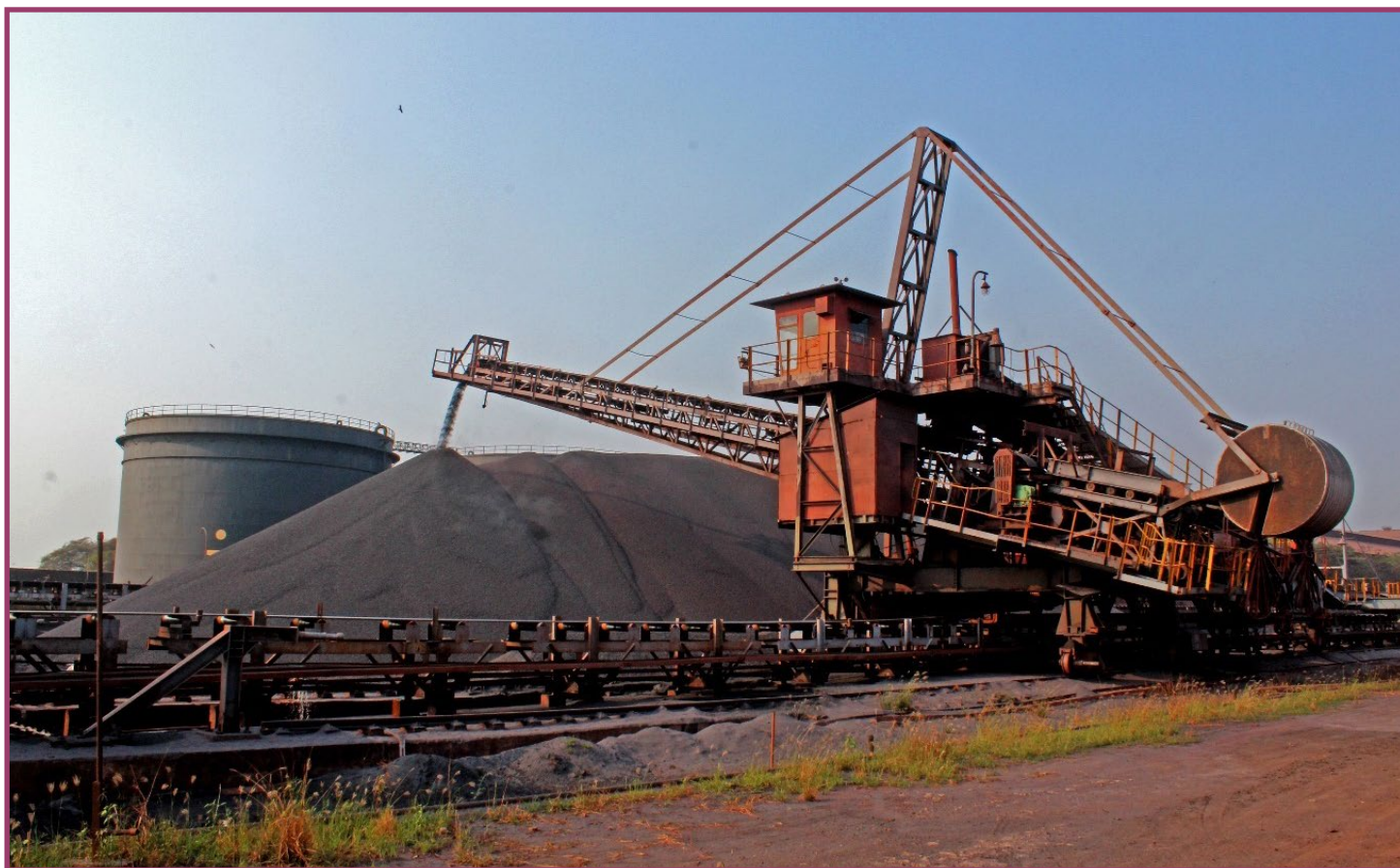
[View of Stacker at Pellet Plant]
