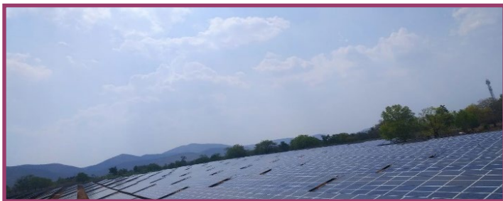
[View of Solar Panels at Kathrikehal]
