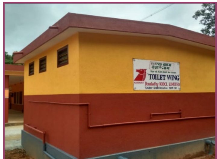
[Urinals and Toilets at at DKZP model Hr. Primary School]
