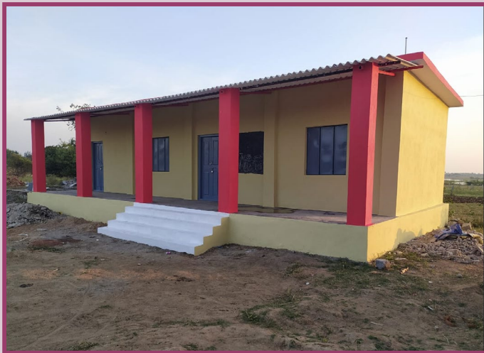
[Two Class Rooms constructed by KIOCL]
