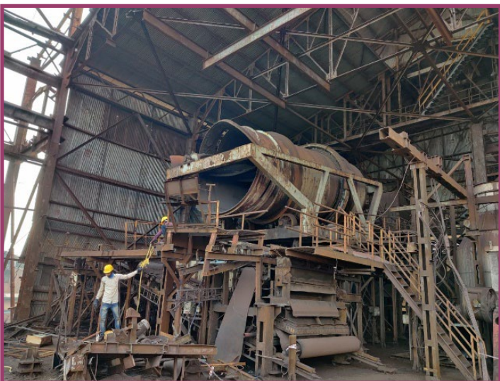
[View of dismantling part of SPF building]
