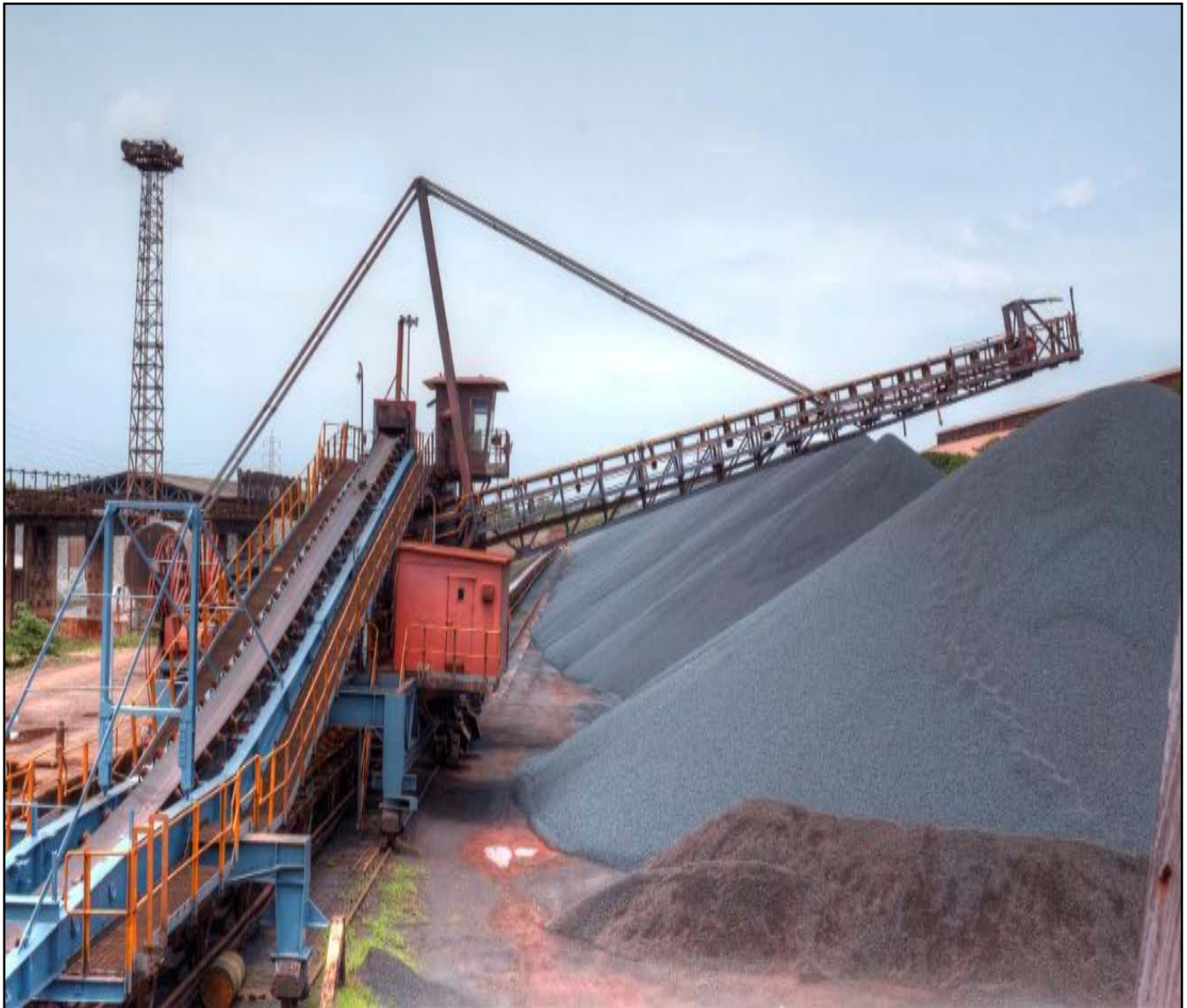
[A view of unloading of Pellets to yard through conveyer belt at Pellet Plant, Mangaluru]
