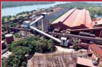
View of Pellet Plant
